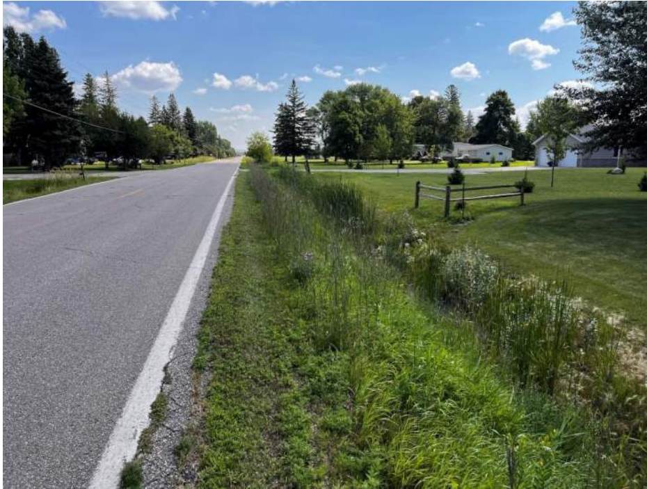
Photo #23. Wet ditch from south ROW 158 th Street, facing east.
