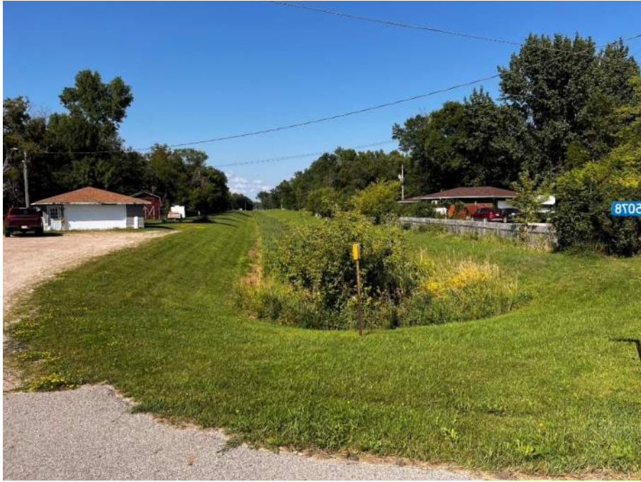
Photo #7. Drainage ditch northwest aspect.
