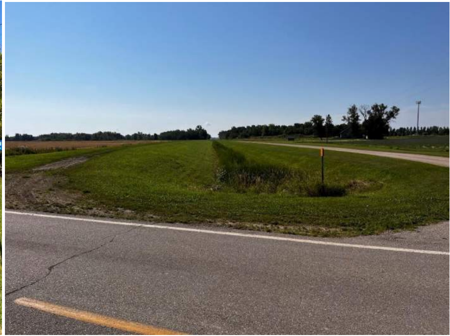
Photo #8. Drainage ditch southeast aspect.
