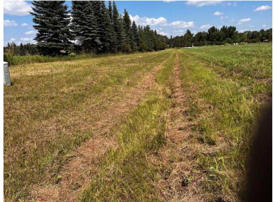
Photo #24. Wet ditch, from west ROW of 150 th Ave, facing north
