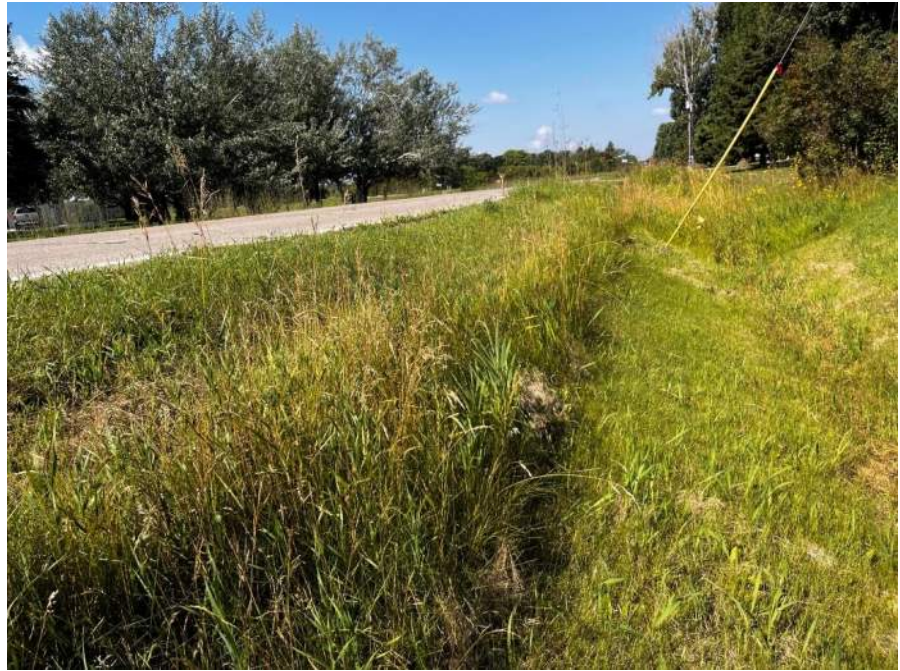
Photo #12 DP 8 facing west. DP7 is located north (right) of image.
